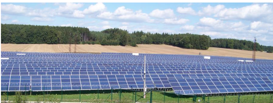
Photovoltaic power plant
